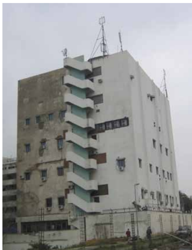
Figure 3. General view of the building
